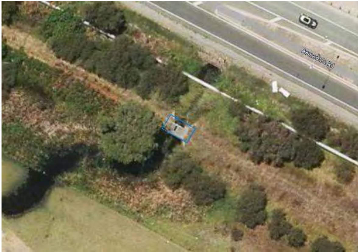
Aerial view of James Drain portion of railway line, with bridge over waterway which runs underneath Armadale Road.
