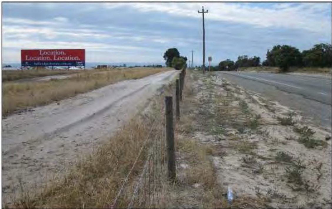
Figure 10: Looking east from corner of Armadale Road and Wright Road along north side of survey area with surface geology typical of survey area.
