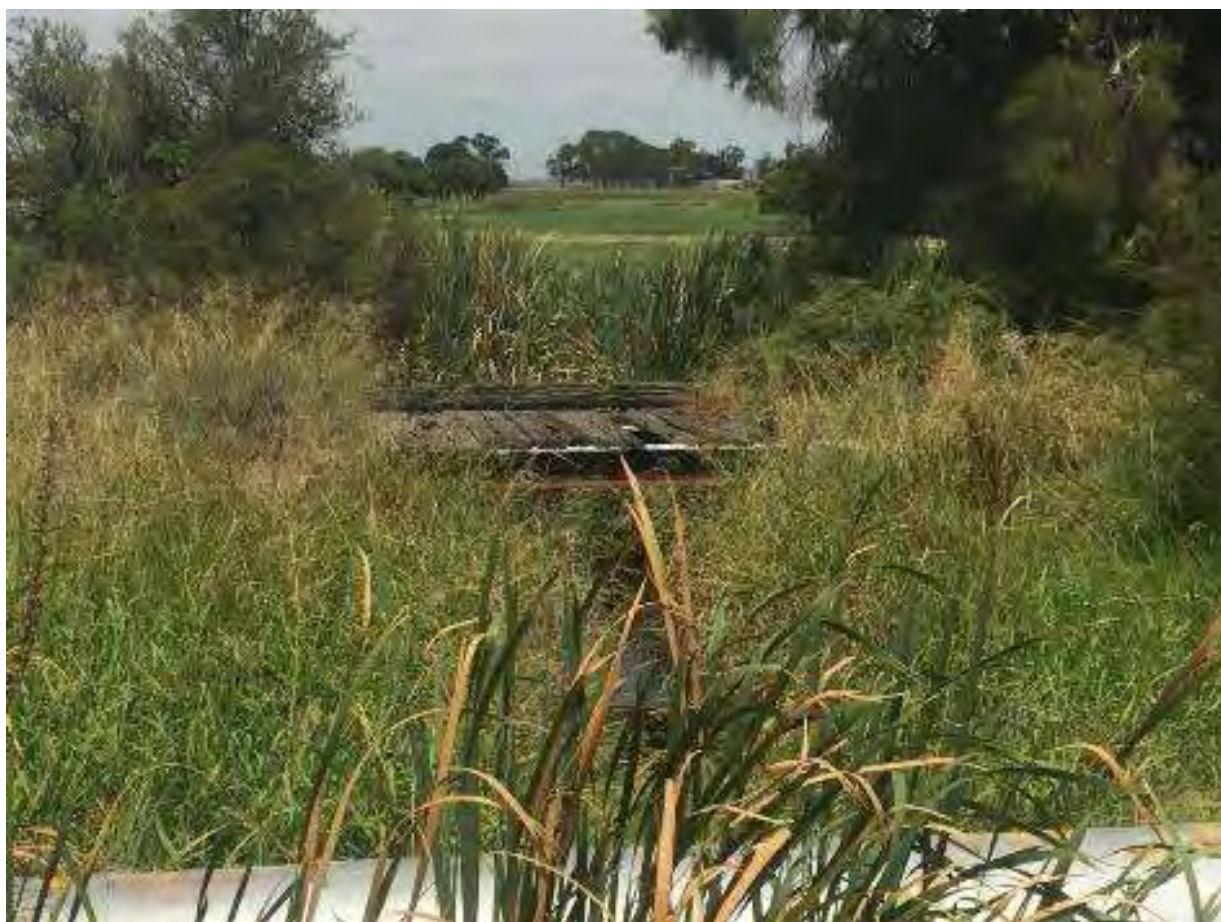
Photo: Bridge at James Drain, Feb 2017.
