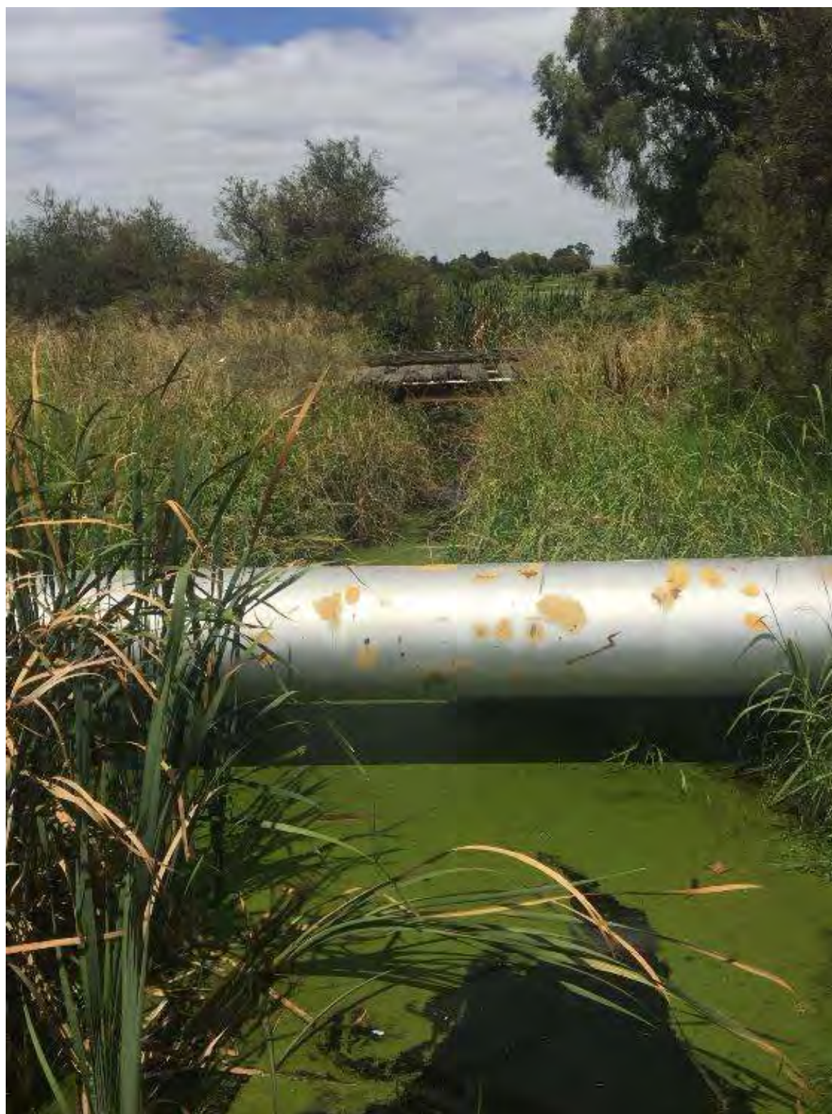
Photo: Water pipeline and bridge at James Drain, Feb 2017.
